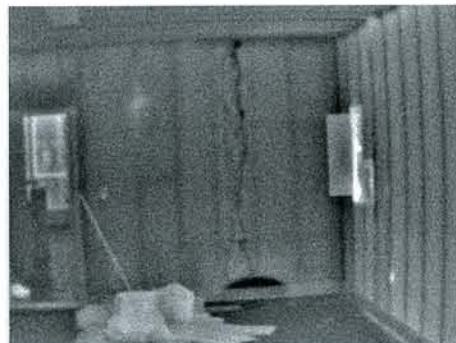
NO SUPERMAN: It's not quite X-Ray vision, but Spencer Maxcy's infrared equipment allows him to see hidden leaks and termite activity in the homes he inspects. An improperly installed HVAC unit leaks into a stud-and-sheetrock wall, but only the IR image (below right) can see it.
